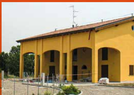
Building constructed with the Isotex® building system
